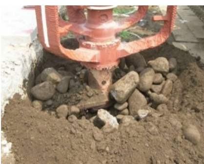
(c)玉石礫質土施工
